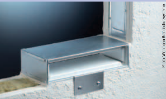
Fire-protected cable bulkhead
